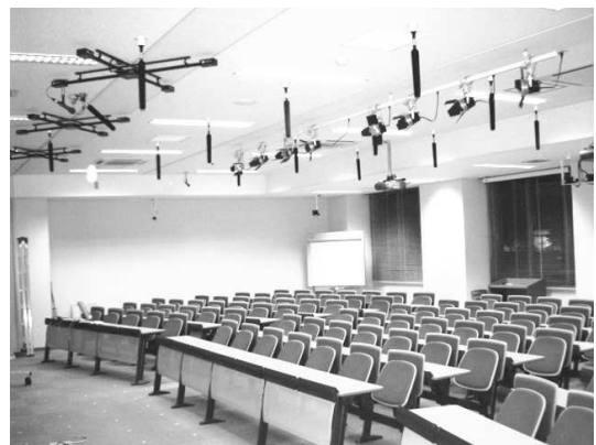
Fig. 1. The classroom at Media Center of Kyoto University designed for distance lectures and equipped with microphones installed over the students area to capture their activity.
