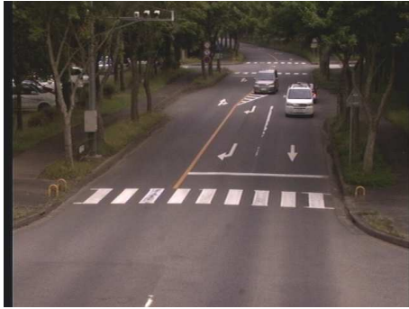
Fig. 9. Surveillance camera image.
